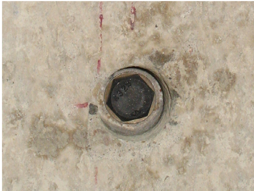
Figure 3.7: Concrete surface after installation of High-Tension Friction-Grip Bolt (HTFGB)
