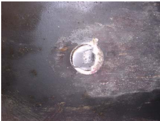
(a) Failed connector in the steel plate
