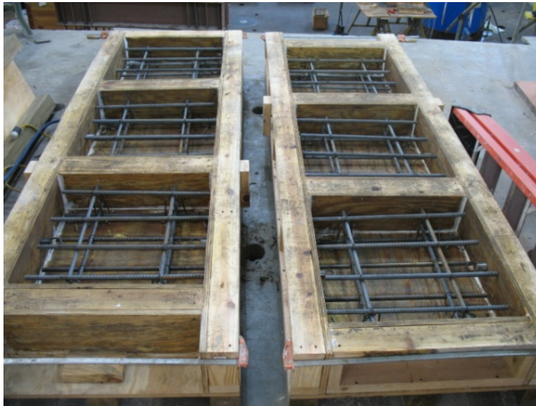
Figure 3.3: Concrete formwork and reinforcing bar layout before concrete casting
