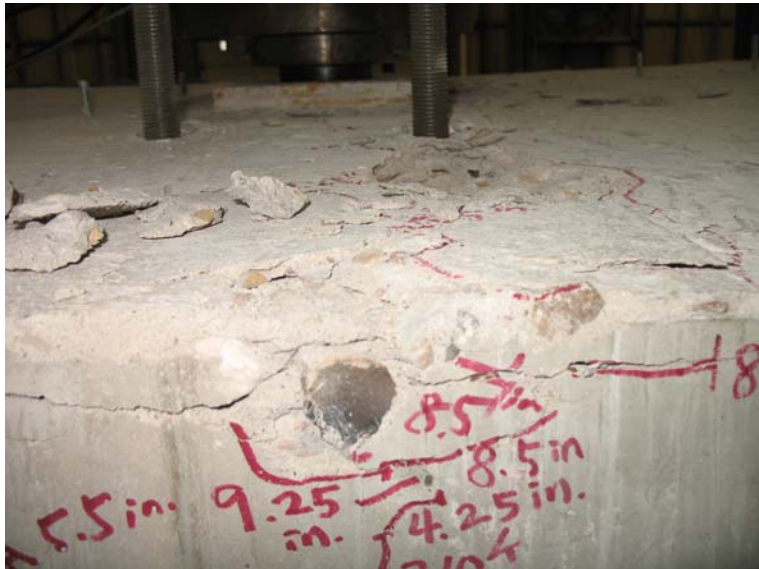
Figure 4.36: Specimen HTFGB-30BS – concrete crushing on the top (10.5-in. deflection)
