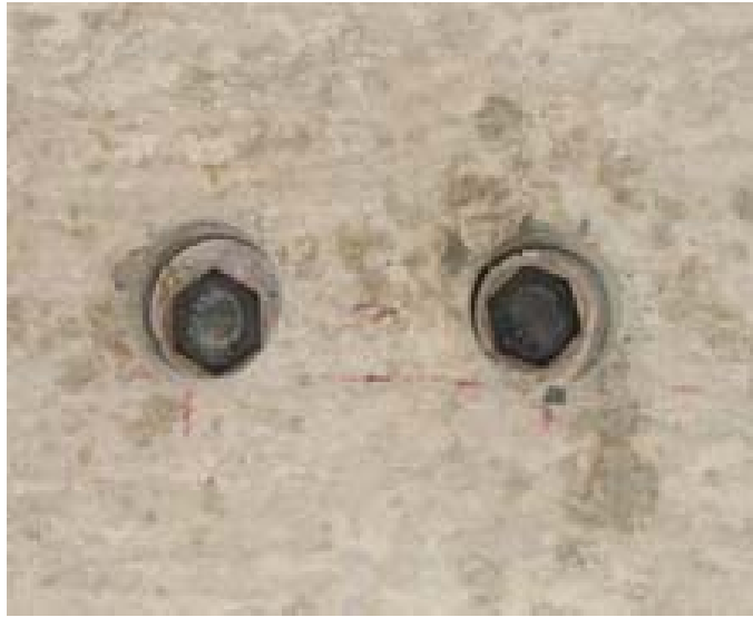
Figure 4.10: Shear connectors installed in hole (HTFGB)
