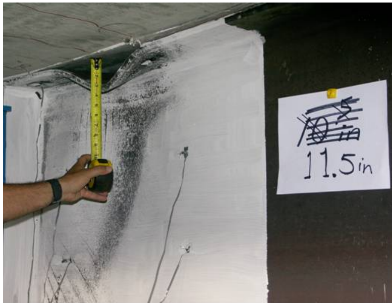
Figure 4.37: Specimen NON-00BS – Typical beam local flange and web buckling at large displacements
