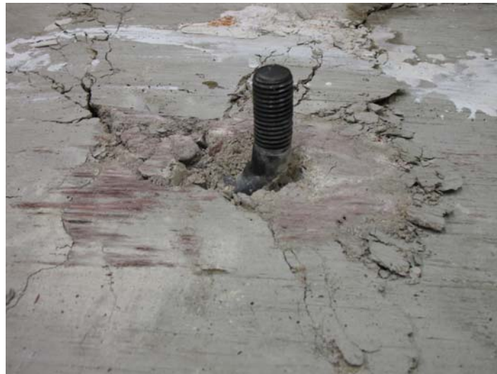
Figure 3.19: Cracks in the concrete block and deformed connector (HTFGB-05ST)
