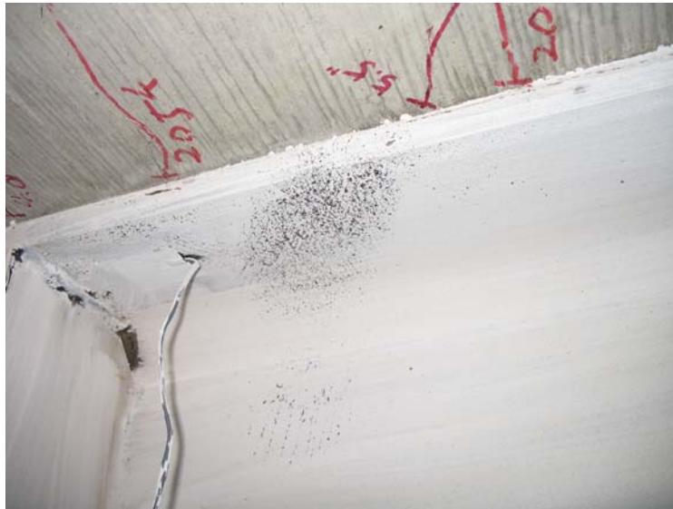
Figure 4.63: Specimen HASAA-30BS1 - Flange white wash flaking (5.75-in. deflection)
