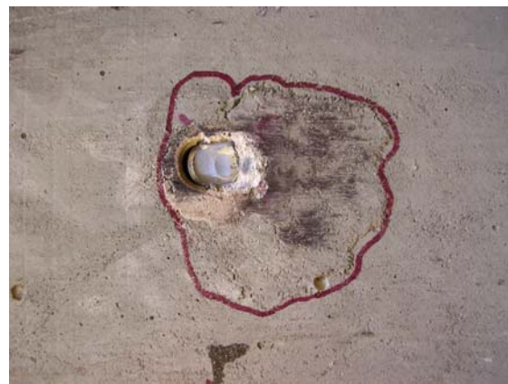
(b) Failed connector in the concrete block
