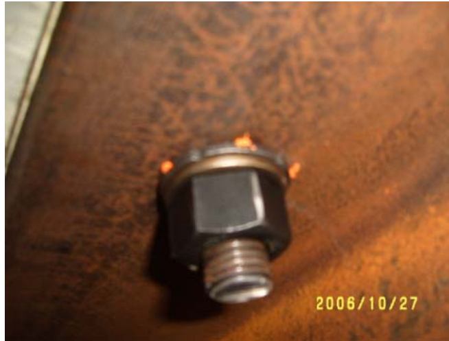
Figure 4.8: Use of “Squirter” Direct Tension Indicating (SDTI) washer
