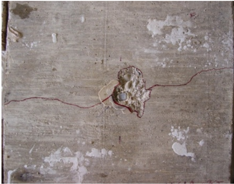
Figure 3.29: Cracks in concrete block (HASAA-12ST)
