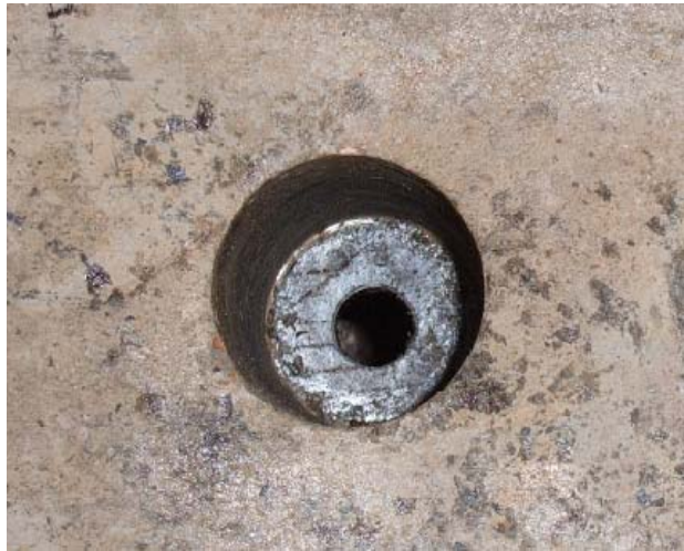
Figure 4.7: Drilled holes for DBLNB installation
