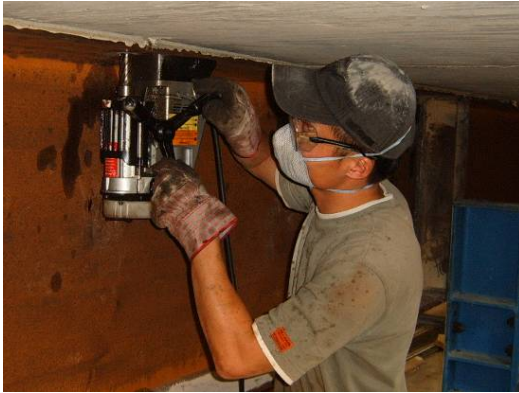
(a) Drilling through the steel flange
