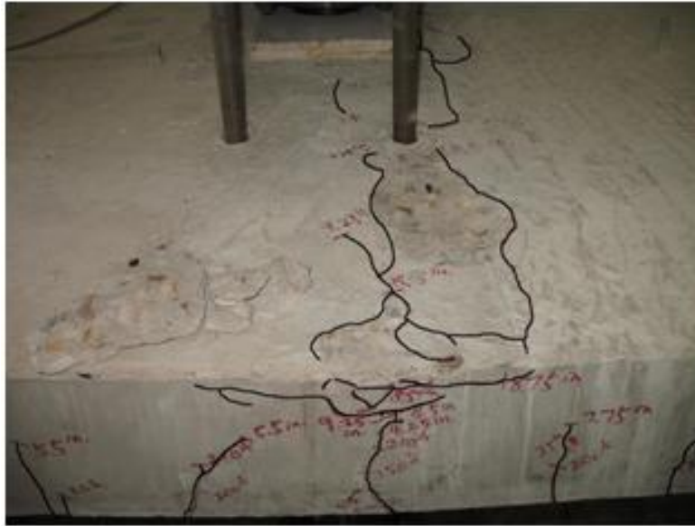
Figure 4.33: Specimen HTFGB-30BS – Concrete crushing on the top of the slab (10-in. deflection)
