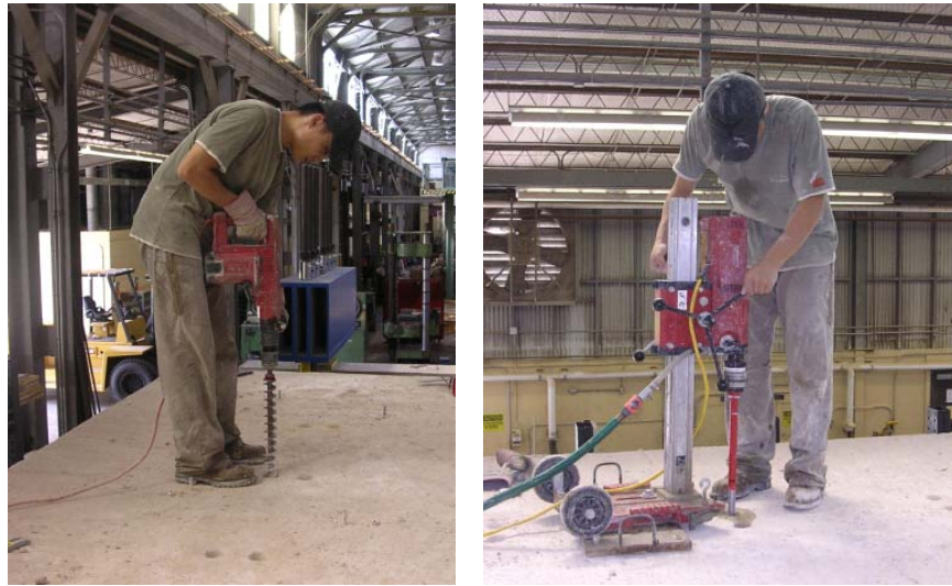
Figure 4.9: Drilling and coring into the concrete slab
