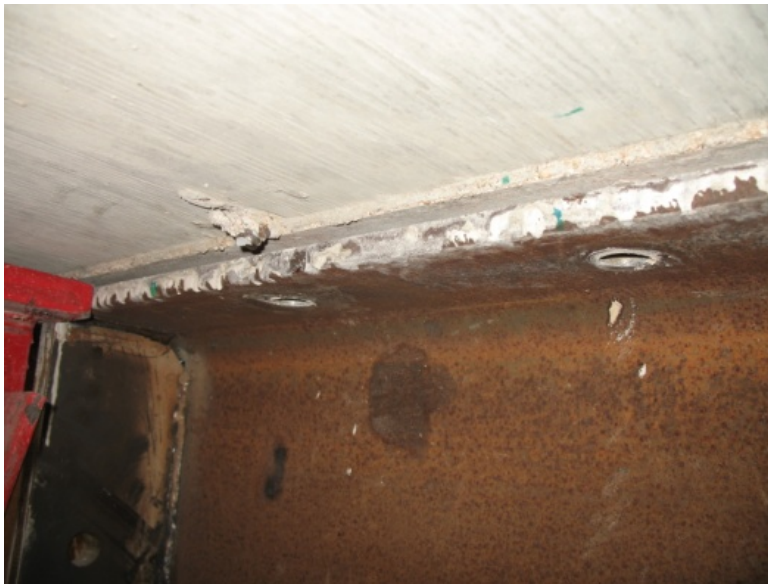
Figure 4.65: Specimen HASAA-30BS1 - Concrete cracks and gap at the interface near the north support (11.25-in. deflection)
