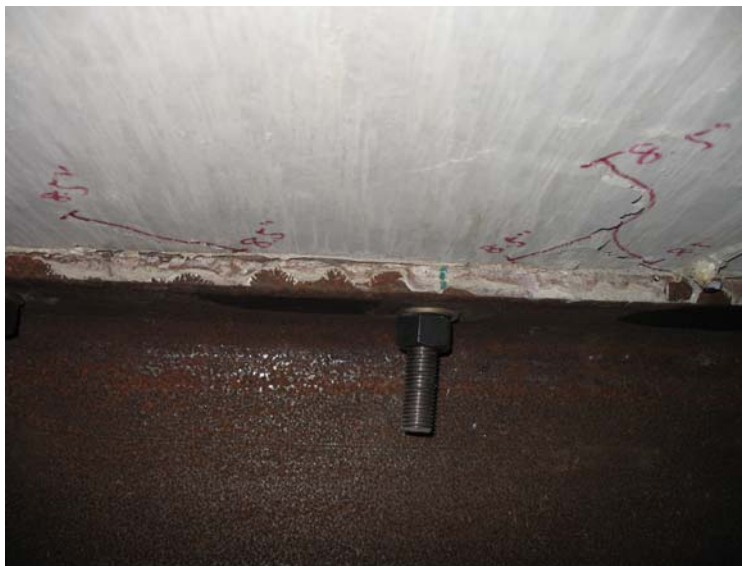
Figure 4.64: Specimen HASAA-30BS1 - Cracks around shear connector (8.5-in. deflection)
