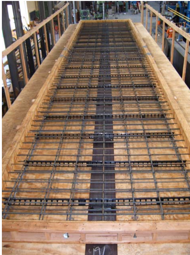
Figure 4.2: Reinforcement layout
