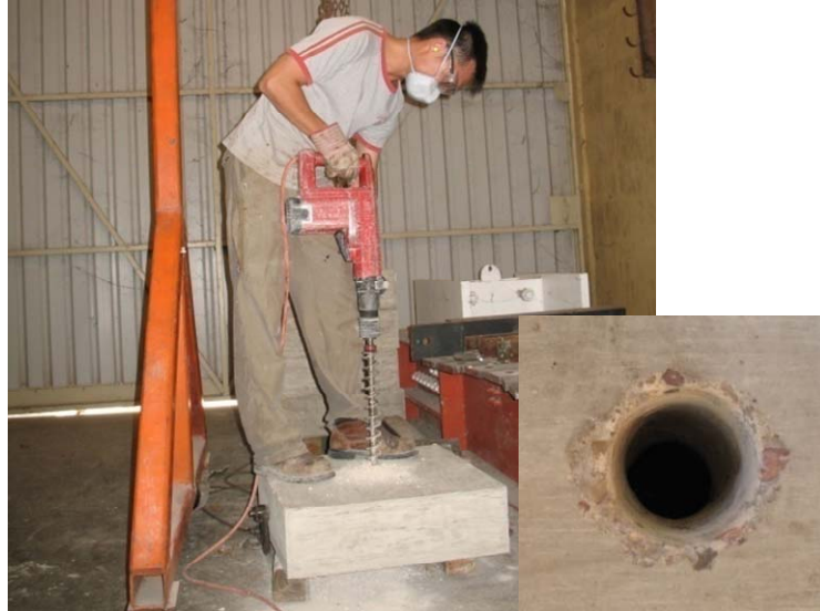
(a) Drilling hole through concrete block
