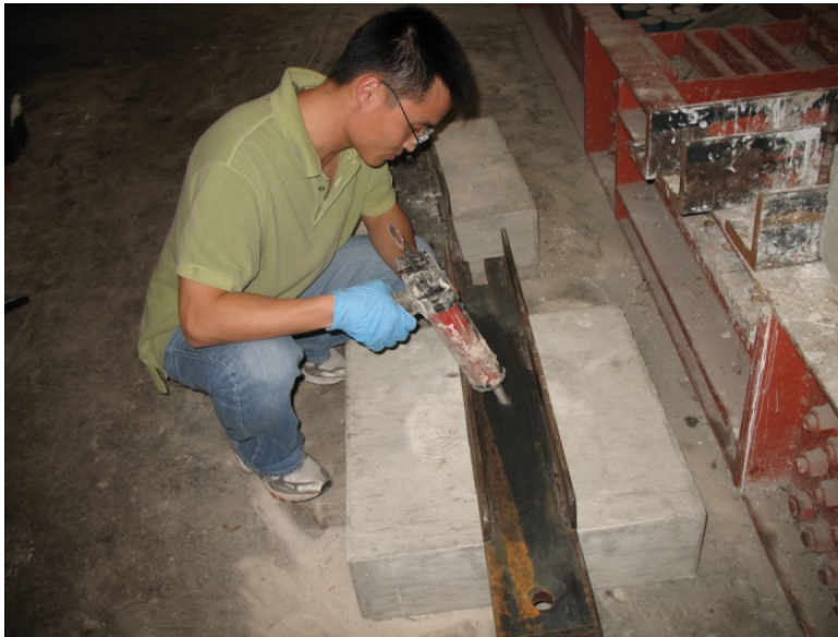
Figure 3.9: Injecting adhesive (HASAA)
