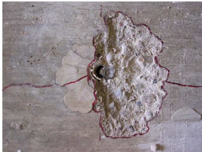
Figure 3.22: Failed shear connector installed in lightly reinforced concrete block (HASAA-11ST)
