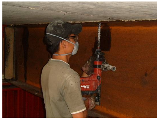
(b) Drilling into the concrete
